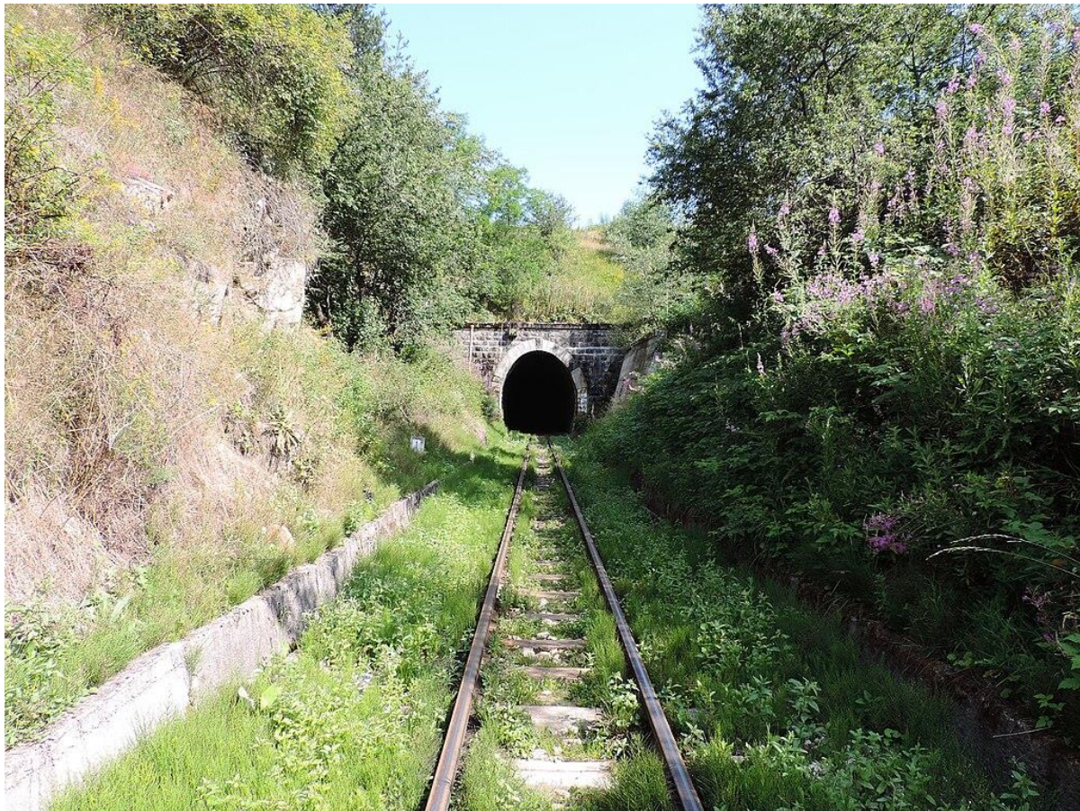
Fig 22. The longest tunnel №32 - 314,26 m. Source: [33]
