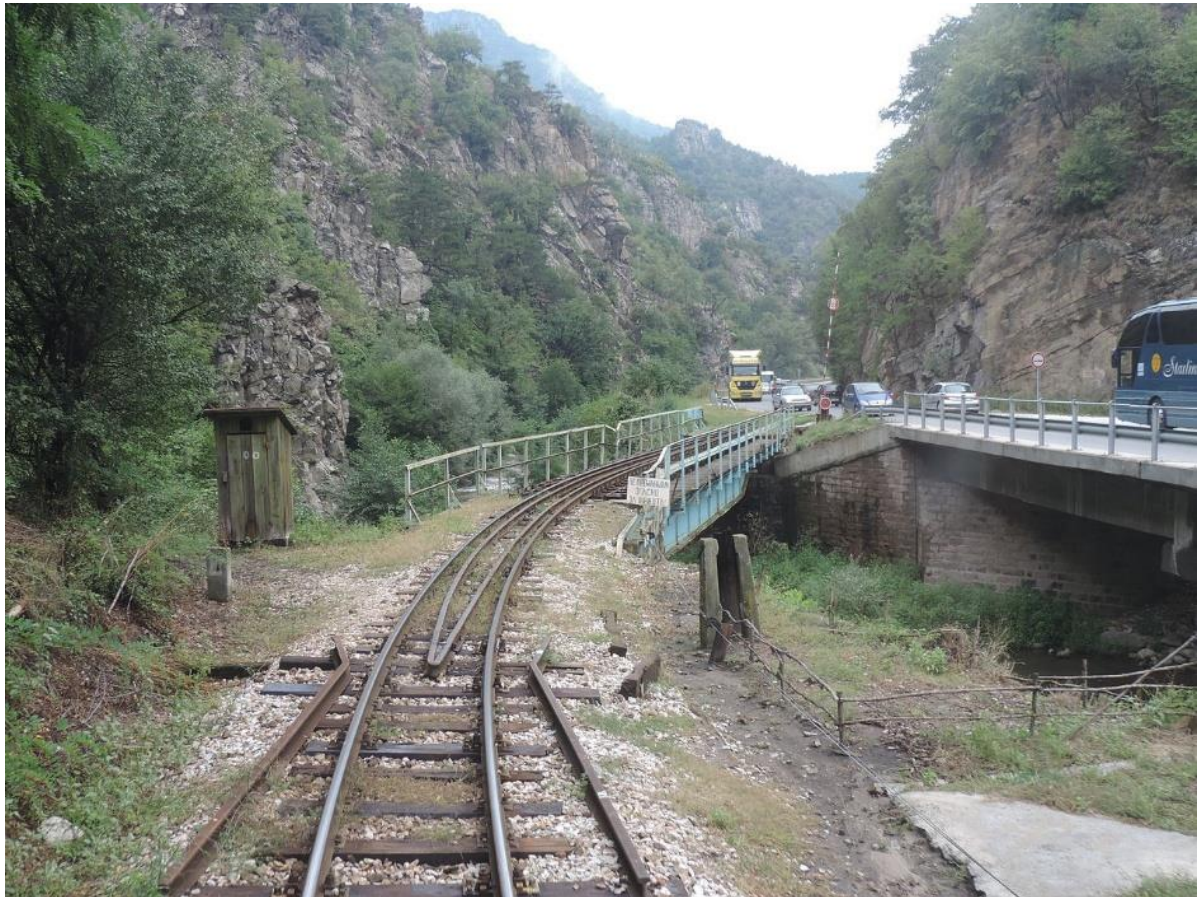
Fig 23. Crossing and bridge over the Chepinska River. Source: [34]
