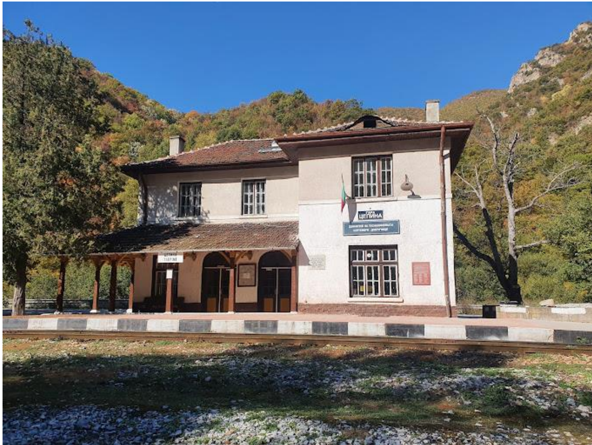
Fig. 4. Train station of Tsepina. Source: [7].
