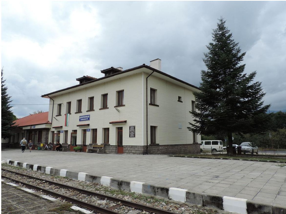
Fig. 8. Dobrinishte station. Source:
